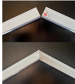
Push both pieces together when installing (the cut piece should overlap the full piece)
