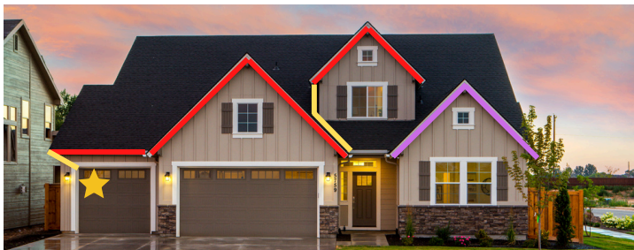
*This is simply an illustration of one potential configuration. Actual placement is subject to personal preference and other physical limitations of your actual property. Diagram for demonstration purposes only. Small to medium sized homes may require only 1-2 runs while larger homes may take 3-4 runs. Note: If the brainbox needs to be placed centrally, the direction for an effect on each run can be reversed in the WLED app if necessary.
